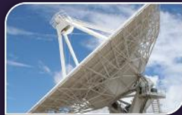
TB Telecommunication & Broadcasting Technology
