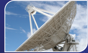
(TB) Telecommunication & Broadcasting Technology
